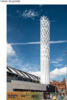
The final sections of Tonkin Liu's 40m-tall biomimetic 'Tower of Light' for Manchester City Council and Vital Energy have been installed.
